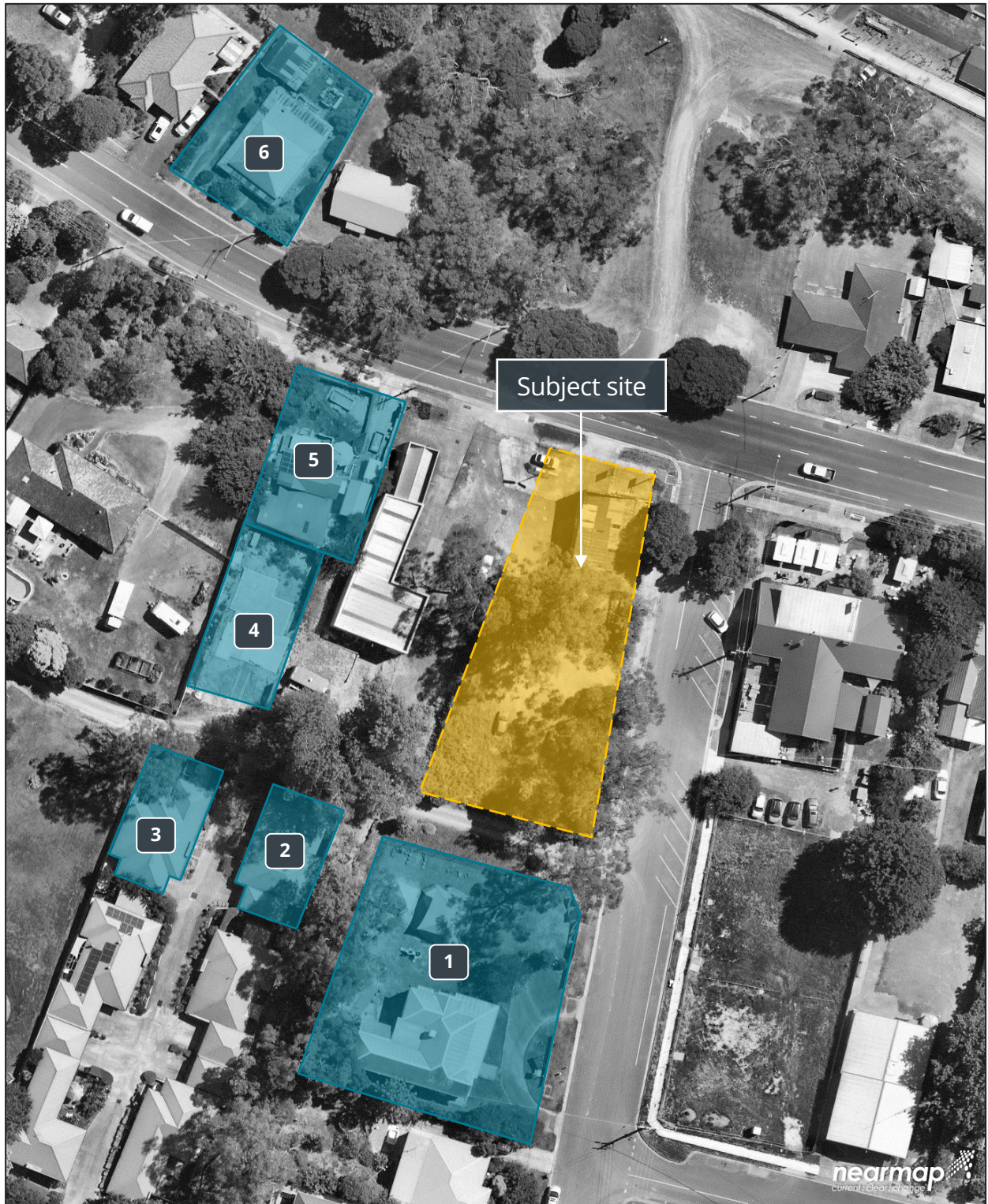
Figure 1 - Aerial photograph of the subject site and receivers (source: Nearmap)
